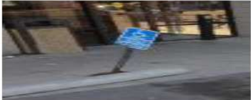
2 – Existing post needs re-erected
