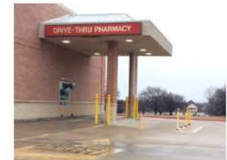
Removed 2 nd lane tube/track system; yellow cone
