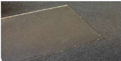
Foot grille fastened to floor on all edges
