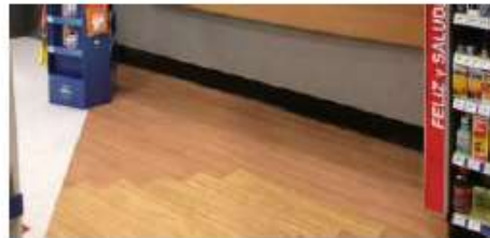
Example of Rx Waiting floor with specification American Cherry, patched with Medium Wood Oak.
