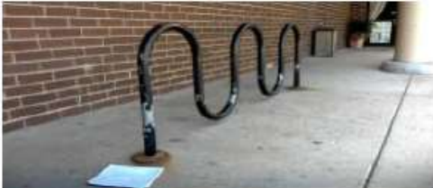
3 – Fixture needs paint/power washed
