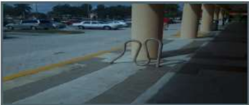
1 – Fixture needs replaced due to rust or damage
